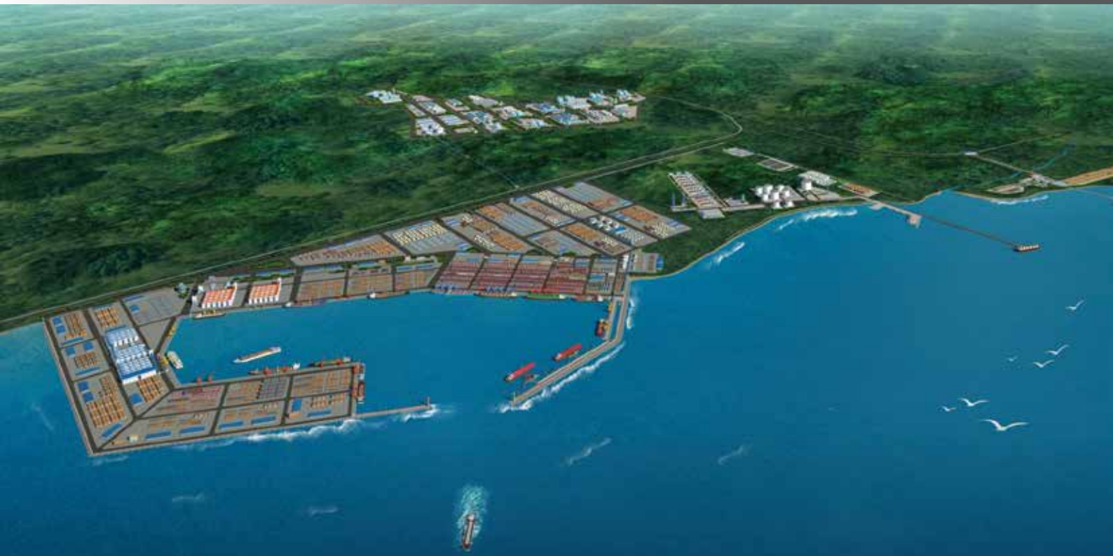
Kribi deep seaport currently under construction by the China Harbor Engineering Company.
